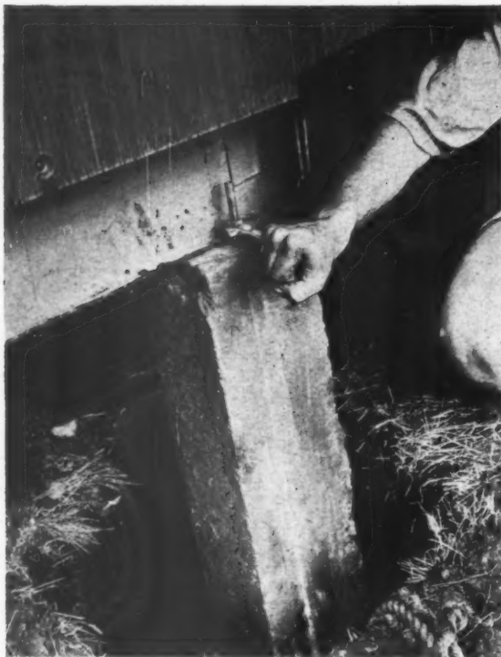
Above, the precast concrete piers being hung from the steel floor beams prior to pouring the concrete footings. Right, fixing the expanded steel ceiling joists to the wall panels.
