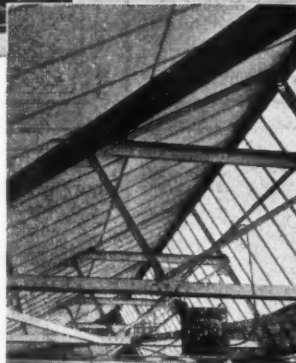
Typical Finish at Ridge on Weaving Shed.
