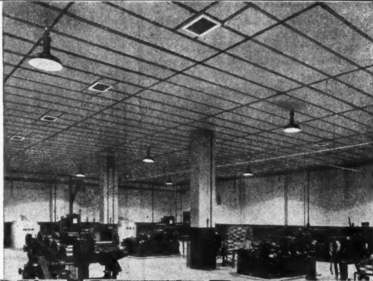
Metal Rolling Mills in the Midland Area showing insulation suspended from Truss Ties
