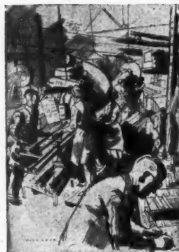
This drawing by Leonard Willcock is the first of a series, "Window Makers at Work" by artists commissioned by Williams & Williams Ltd. It shows the first stage—the cutting and despatch to welders of rolled steel sections for frames.
