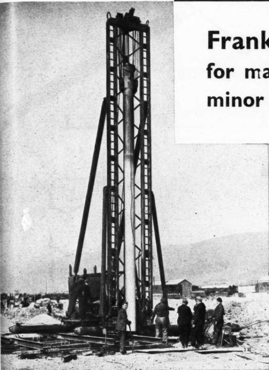
A FRANKI DIESEL MACHINE AT WORK
