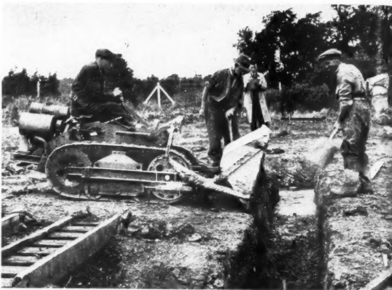
Modified horticultural tractor with aluminium alloy skip discharging concrete into a foundation trench.
