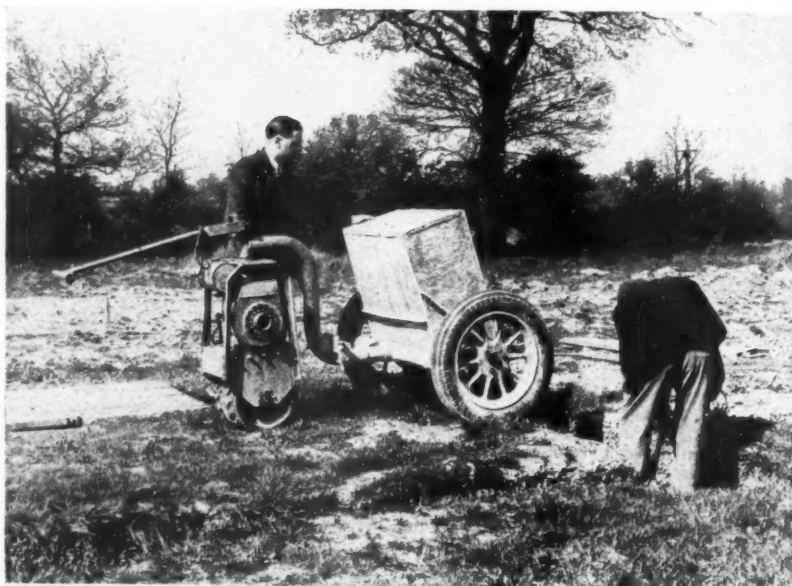
MOW 3-wheeled motorized barrow discharging concrete into trench.
