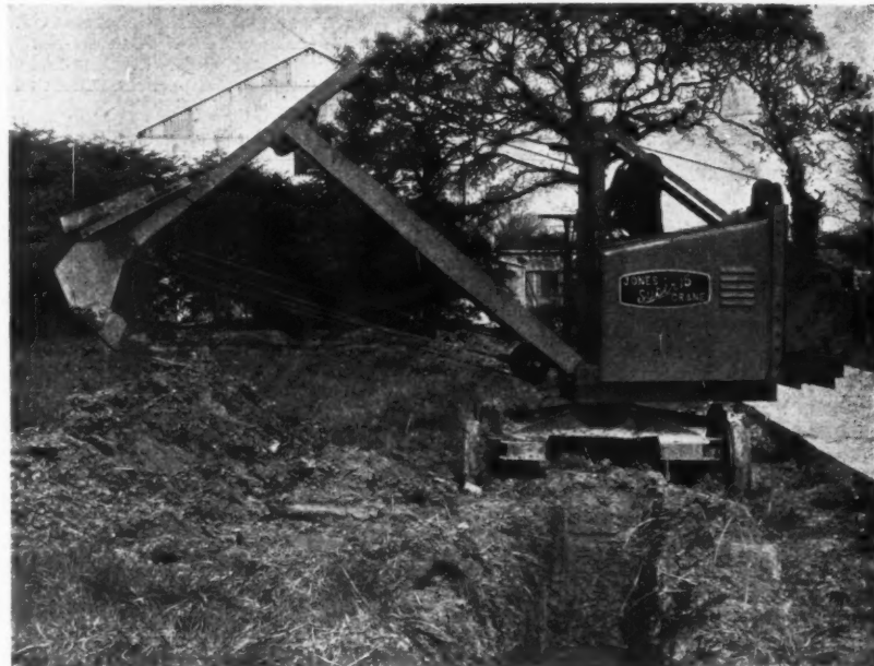
MOW back-acting excavator digging a 22-in. wide trench.
