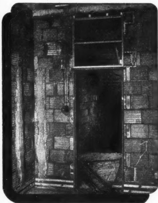
Cranham Terra Cotta Hollow Partition Blocks were specified for the offices of the Bristol Steam Navigation Co., Prince Street, Bristol. ARCHITECT: Eustace H. Bulton, Esq., F.R.I.B.A. CONTRACTORS: C. A. Hayes & Sons, Ltd.
