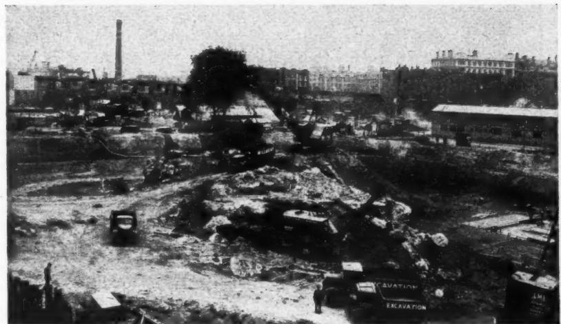
Top, the site in its original water-logged state, showing the dewatering header main and the wells in position. On the right, their roots covered by tarpaulins, are the two trees which are being preserved. Above, excavation in progress. The mass of concrete in the centre is the foundation to the old Lion Brewery.
