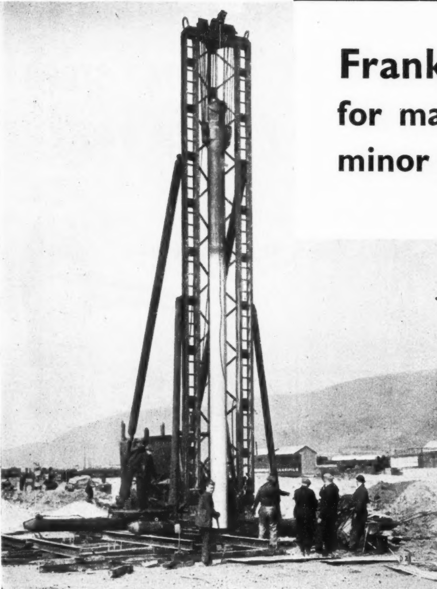
A FRANKI DIESEL MACHINE AT WORK
