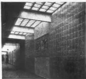
Wide joint tiling in one of the school corridors. The panels of Tiling are in different colours : red, brown, grey and white
