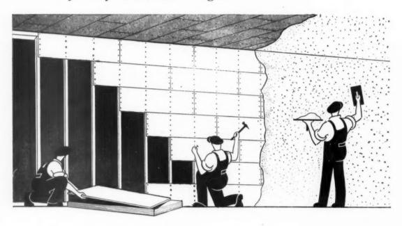
"Gyproc" Lath is an ideal plastering base for "Gyproc" Gypsum Plasters—their combined use minimises the incidence of cracking in finished plasterwork.
