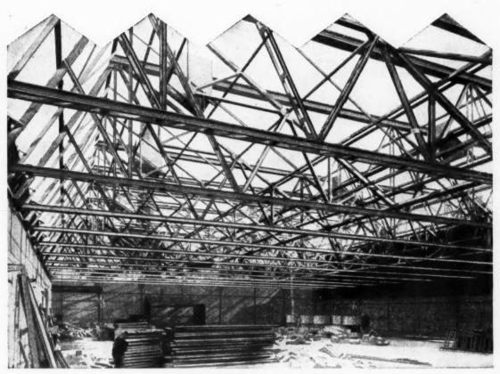
Warren girder roof, 85 ft. clear span
