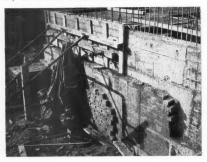
ROOF 2 outer last 12" Carriey, 6" inner head. Weight of outer last transmiller through inoutated dwarf walls to inner leaf
