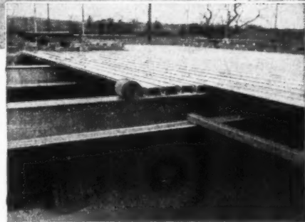
General view of installation of Briggs Bitumetal Roof showing Aluminium Deck Units. The underside presents a clean, attractive ceiling.
