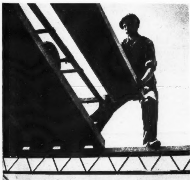
Above, a typical section of the Dow-Mac precast concrete roof beam. Left, a beam being placed in position.
