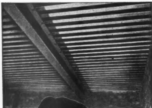
Ceiling effect of "BITUMETAL". Note high reflective value.
