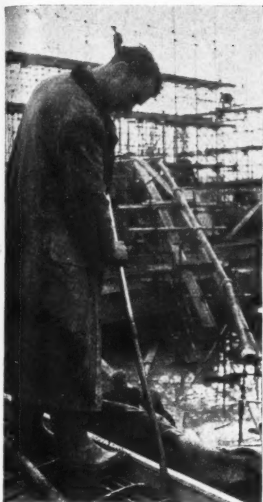
Above, left, cleaning the shuttering with compressed air. Top right, pouring hand-mixed concrete. In the foreground is a pump operating one of the internal vibrators. Above, right, the scale readings for fine and coarse aggregates on one of the batchers. Below, two of the numerous wood box inserts forming openings for service pipes.
