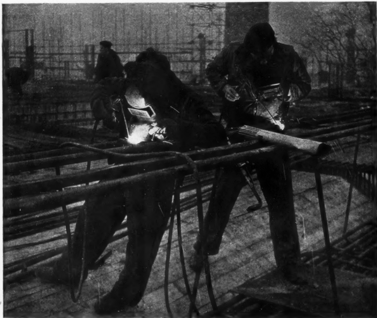
Welding some of the reinforcing bars of large diameter.
