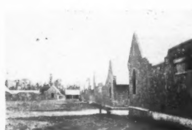
8. Houses for Northern Moslem students, at Vom. The houses are laid out in compound form. Construction is of local stone with dressed copings, etc. Openings in the external walls are kept to a minimum.
