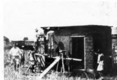
14. Mud block work in course of construction at Ibadan. The foundations are of sandcrete block and the concrete is taken through the external wall as an anti-termite barrier.
