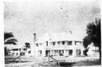
10. A house for a European Civil Servant, Ikoyi, Lagos. Walls are of sandcrete block, ground floor of concrete, first floor of timber, roof of corrugated asbestos.
