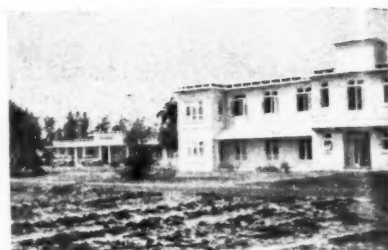
13. Flats at Ikoyi, Lagos. The double roof, consisting of precast concrete slabs placed on the main roof, adds a considerable superimposed load but is an efficient and cheap method of insulation.
