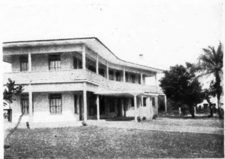
12. A house for the manager of a commercial company, Ikoyi, Lagos. A most successful design, careful attention having been given to the detailing of the balcony, overhanging eaves and entrance porch.
