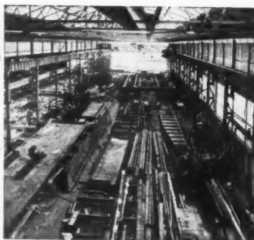
View of our heavy fabricating bay showing typical heavy riveted girder work.
