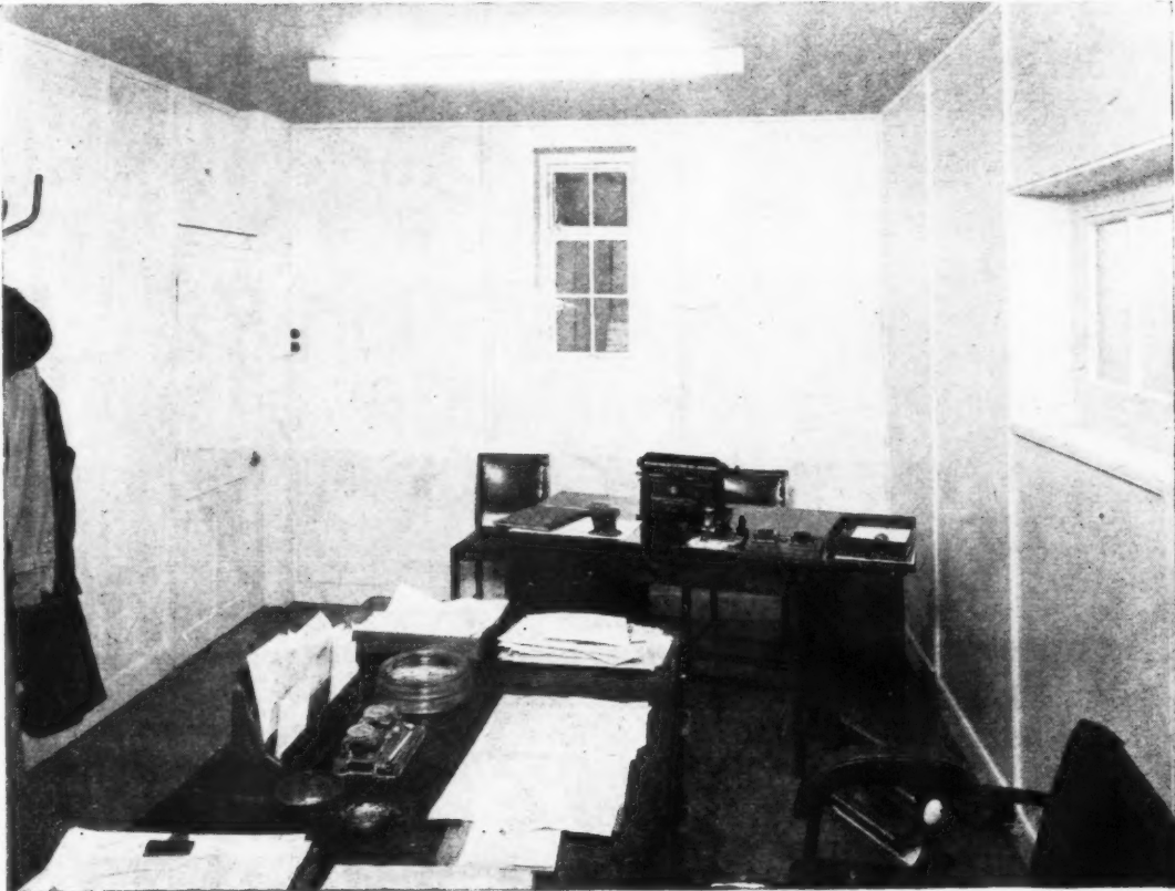
The above illustration shows the conversion of offices, ceiling and walls having been clad throughout with \frac{1}{2} in. PLIMBERITE and the partition was constructed with \frac{3}{4} in. PLIMBERITE.
