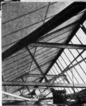
Typical finish at ridge on Weaving Shed.
