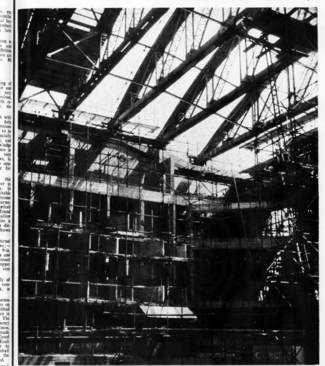
Inside the auditorium. The side walls are complete, the inner skin of the roof is being laid and the casting of the balcony is in progress.
