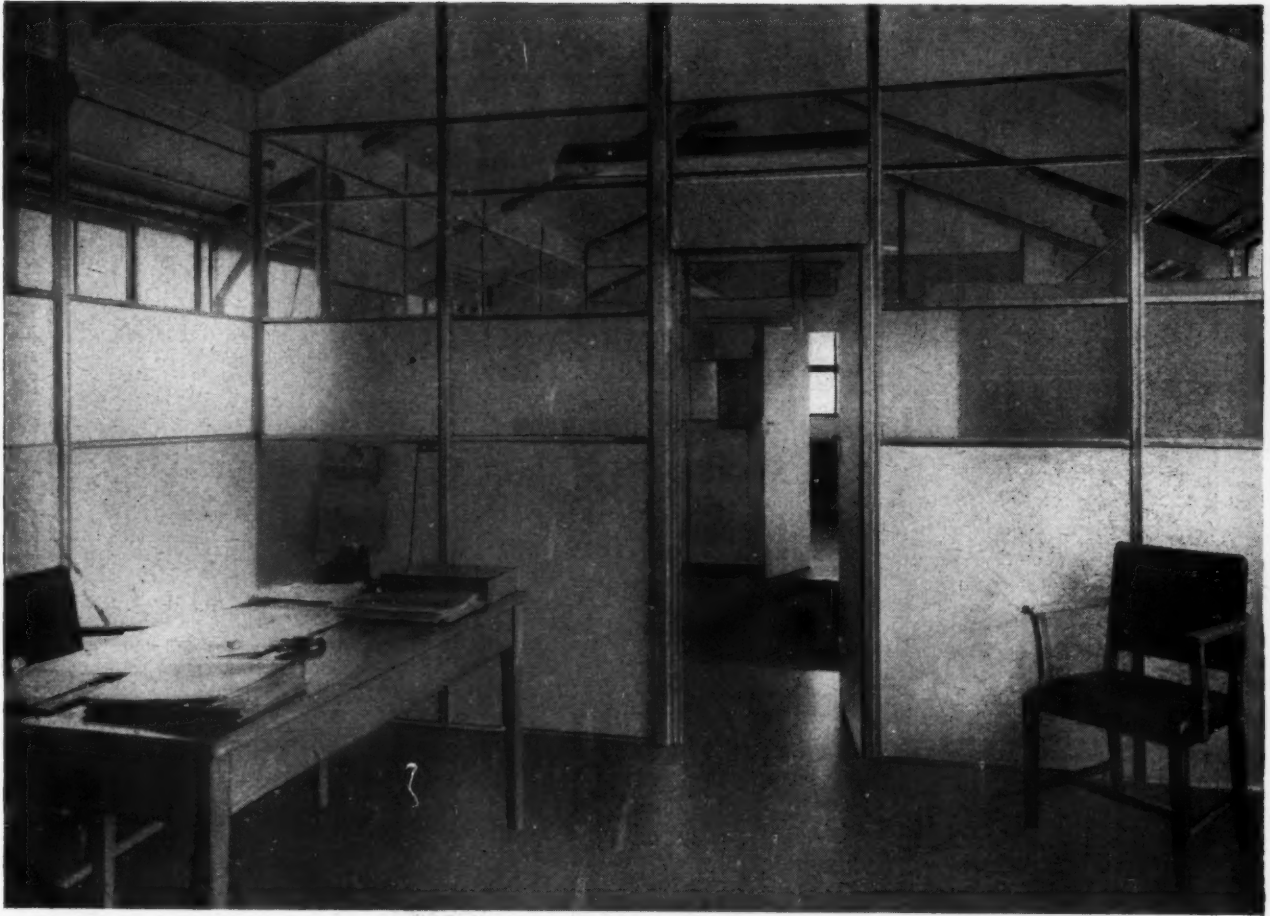
General view of offices of K. L. M. Royal Dutch Airlines, at London Airport, designed by J. Stroud Foster, A.R.I.B.A. Conversion of concrete hut executed by Compactom Ltd., with partitioning of "PLIMBERITE" and glazing in aluminium framing.
