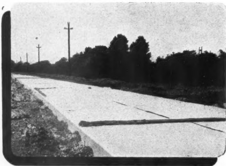
Typical example of a concrete road slab blanketed with Sisalkraft.
