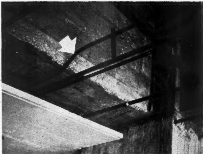
Above, typical steel hangers and fibrous plaster ceiling clothing the concrete structure. The arrow indicates an electric conduit running in the cavity.
