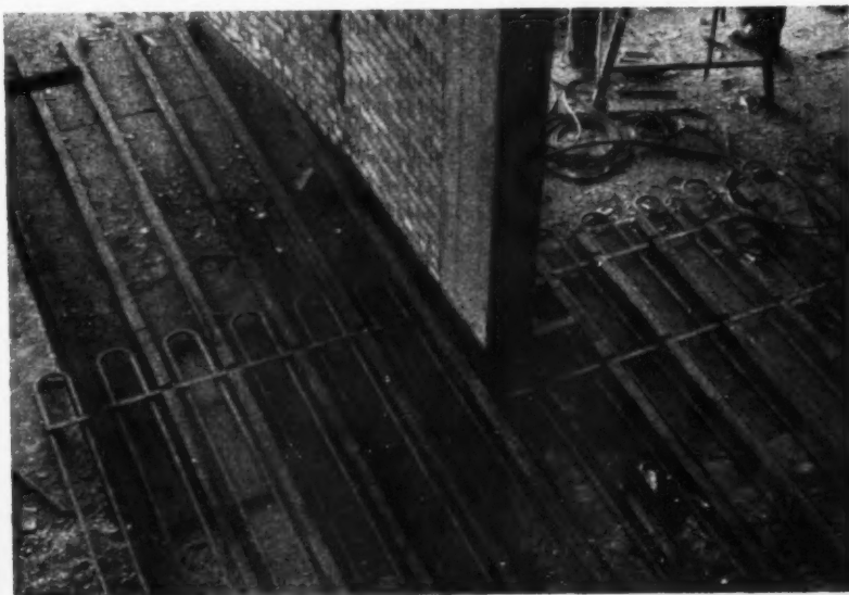
Above left, a pair of flow and return HW heating pipes serving a number of distribution pipes. Above right, recently fixed fibrous plaster ceiling to foyer, showing extract grilles and lighting troughs. The opening in the bottom left-hand corner is for a tungsten fitting. Below, typical flow heating panel in steel tube, showing cork insulation beneath and battens on clips for strip flooring.
