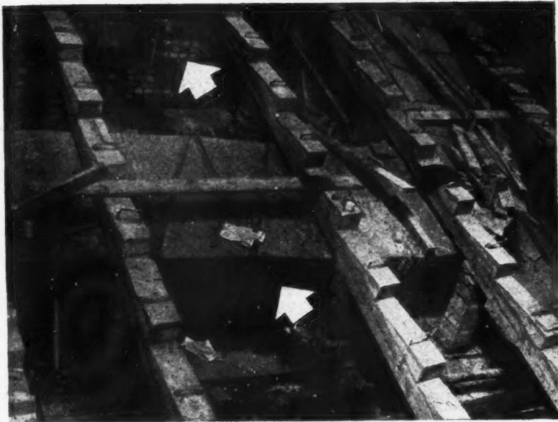
Above, extract ducts beneath the auditorium stepped floor. One of these ducts is formed of brickwork rendered internally and the other of galvanized steel. Brickwork was used for economy where there was room.
