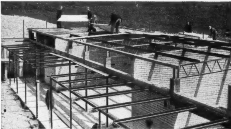
This photograph shows STRAMIT roofing slabs (4ft. by 8ft. 3in.) being laid to form a decking for bituminous felt at Elaine Avenue Primary School, Strood, Kent. (Architects: Messrs. Moiret & Wood, A.R.I.B.A., London in collaboration with S. H. Loweth, Esq., F.S.A., F.R.I.B.A., County Architect. Roofing Contractors: Neuchatel Ashphalte Co. Ltd., London. General Contractors: Kent & Sussex Contractors Ltd., Sidcup, Kent. Special purlins to the registered design of Messrs. Moiret & Wood).
