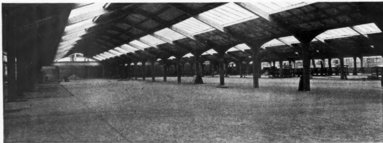
A New Factory for the Morgan Crucible Co. Ltd., engaged in the manufacture of high grade refractories. Concrete floors treated with EVODE PROVER II CRYSTALS for hardening and dustproofing. General contractors: Messrs. A. Monk & Co. Ltd. Civil Engineering & Building Contractors, Padgate Warrington.
