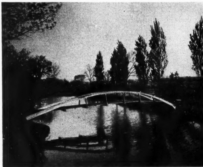
This wooden footbridge near Princeton, New Jersey, is included in "The Architecture of Bridges", reviewed on this page. It was designed by Kenneth Kassler, architect and Kraemer Luks, engineer. The tapered curves of the fixed arches are a lucid expression of the transfer of weight and thrust to the concrete abutments.
