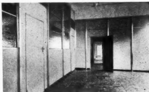
General view of City Offices showing glazed Corridor Partitions 12' high with inter-communicating doors through transverse solid Partitions. Aluminium Junctions and Partitions with 1" cream painted panels.
