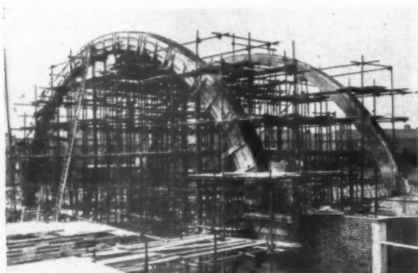
First rib complete, shuttering erected for second rib.
