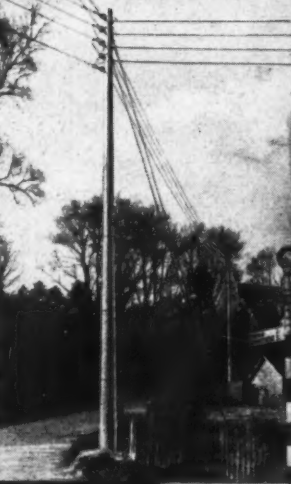
L.T. DISTRIBUTION STAYED JUNCTION POLE
