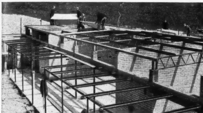
This photograph shows STRAMIT decking (4ft. by 3ft. 3in.) being laid to form a decking for bituminous felt at Elaine Avenue Primary School, Strood, Kent. (Architects: Messrs. Moiret & Wood, A.R.I.B.A., London in collaboration with S. H. Loweth, Esq., F.S.A., F.R.I.B.A., County Architect. Roofing Contractors: Neuchatel Asphalte Co. Ltd., London. General Contractors: Kent & Sussex Contractors Ltd., Sidcup, Kent. Special purlins to the registered design of Messrs. Moiret & Wood).
