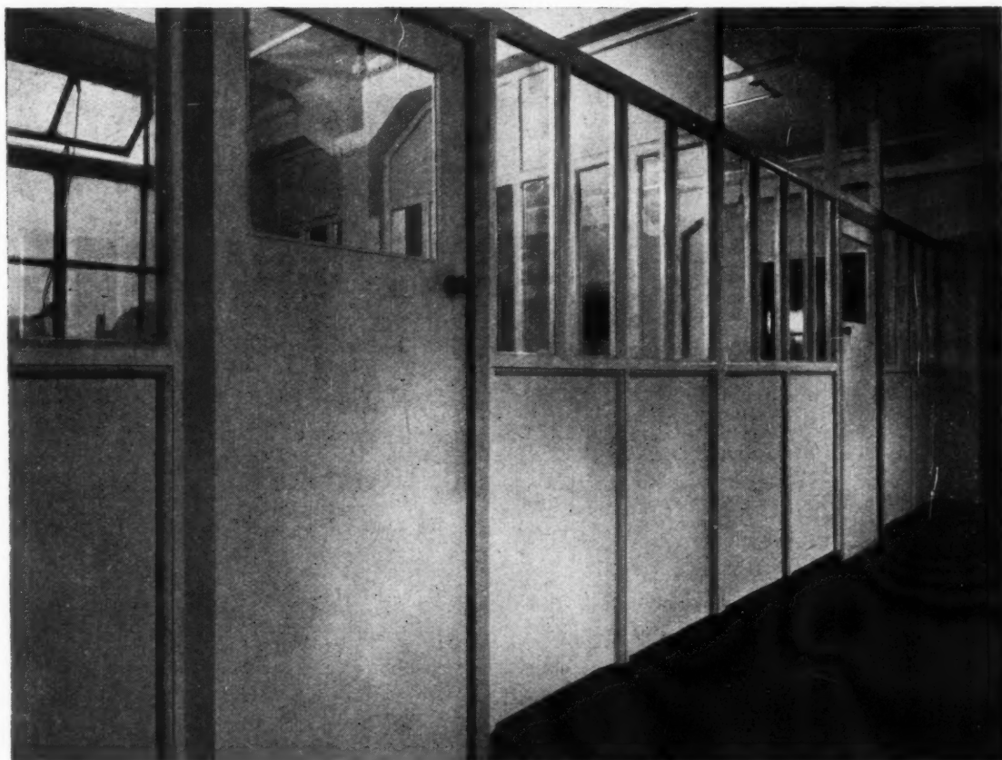
Office partitioning constructed with \frac{3}{4} in. PLIMBERITE and timber framing, work having been carried out by Messrs. Batger & Co., Ltd., Confectionery Manufacturers, 566 Cable Street, Stepney, London, E.1, to their own designs at their Cable Street Premises.
