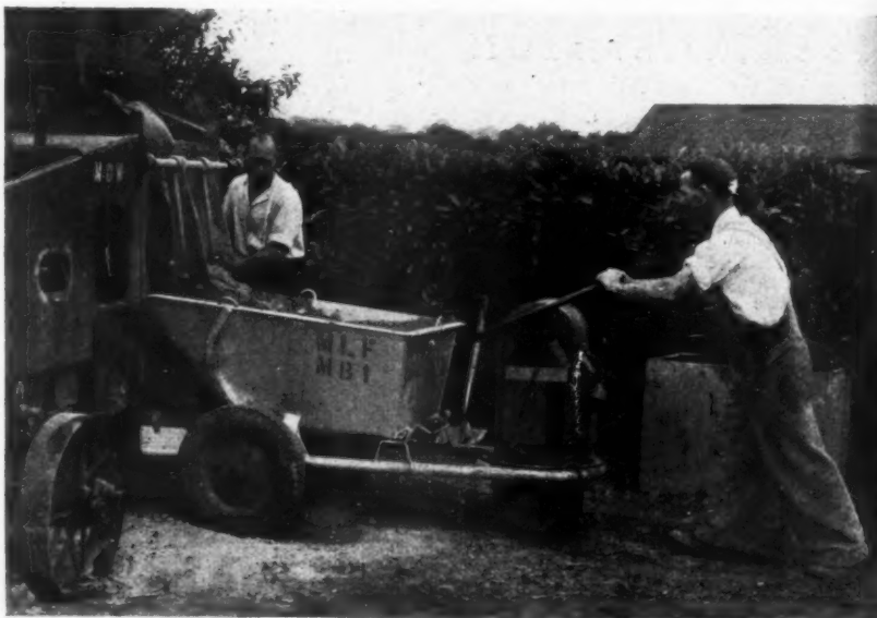
Above, Fig. 3, typical powered concrete barrow; below, Fig. 4, Single rail concrete transporter.
