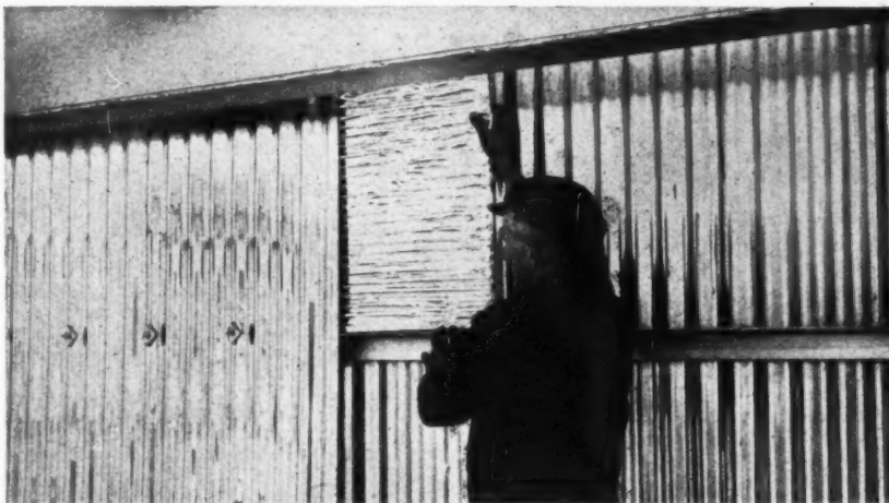
Tucking insulating foil packs behind a freshly applied aluminium sheet on the inner wall.
