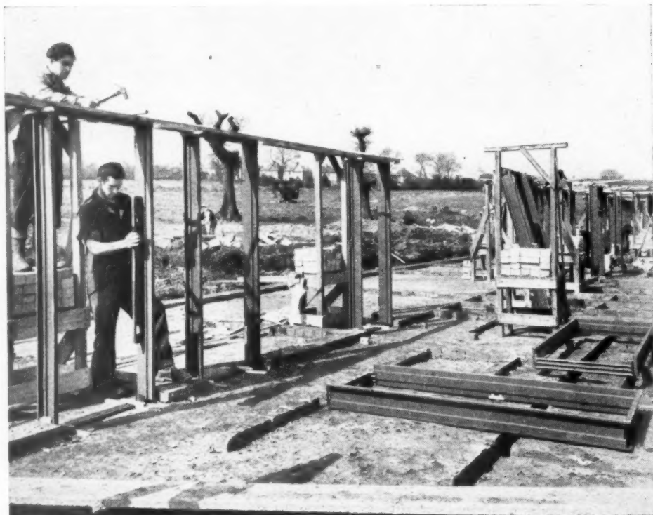
PLUMBING & STRUTTING DOOR FRAMES FOR A BLOCK OF FLATS
