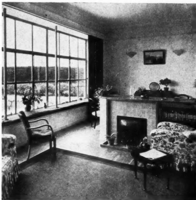
The lounge and dining space beyond. The purpose made 22-ft. by 7-ft. 8-in. steel window is set in a reinforced concrete surround which has been poured in situ.
