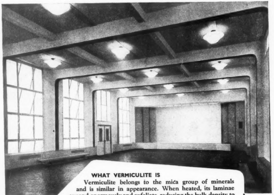
"Kisol" Vermiculite Plaster for inside wall and roof treatment for London County Council School.
