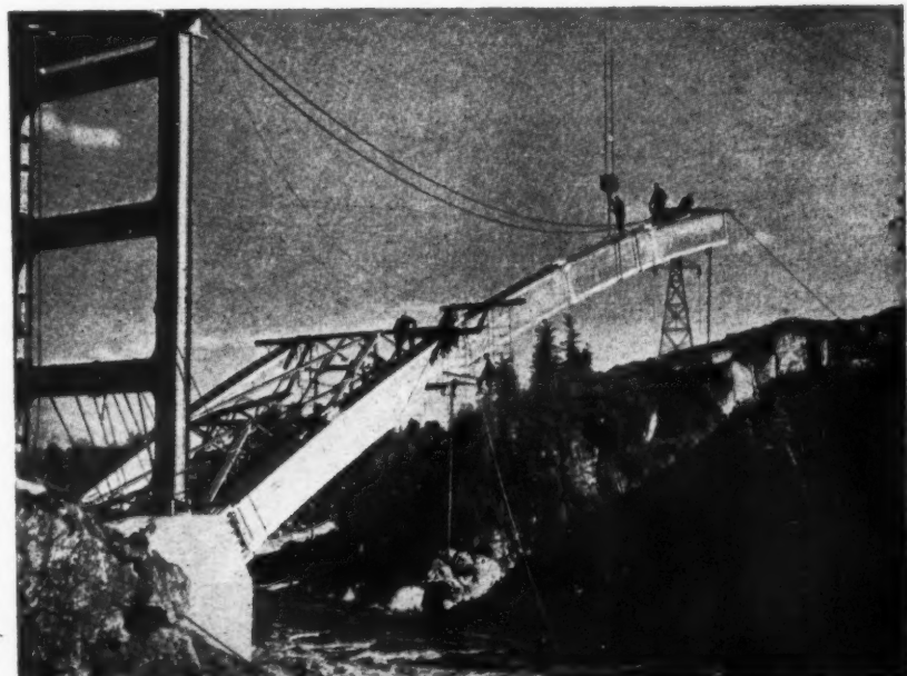
Aluminium arch bridge, being erected by cantilever method. See 20.189.
