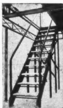
Built at Mills' Birmingham Depot. A prefabricated staircase, easy to handle yet stout and rigid.
