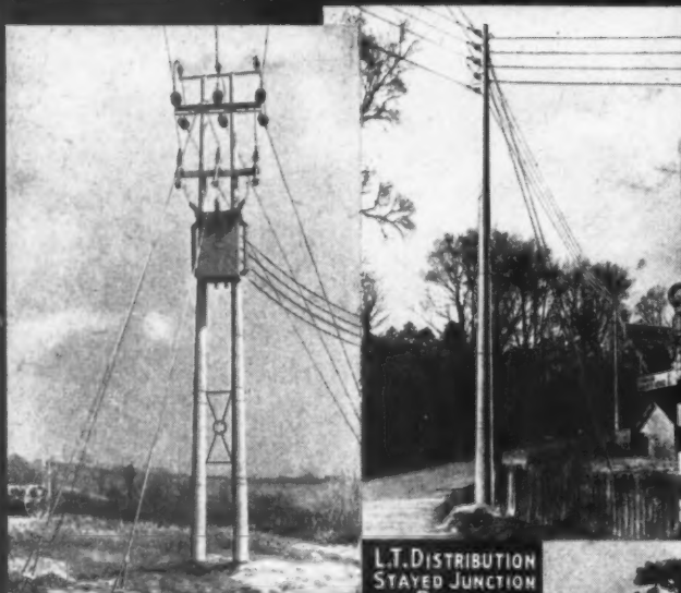
6.6 K.V. OVERHEAD LINE TRANSFORMER STRUCTURE
