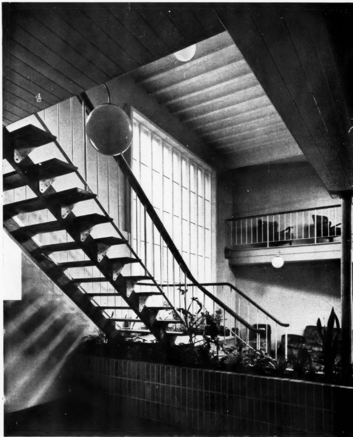
The staircase treads are of hardwood carried on aluminium alloy brackets fixed to timber carriage beams
