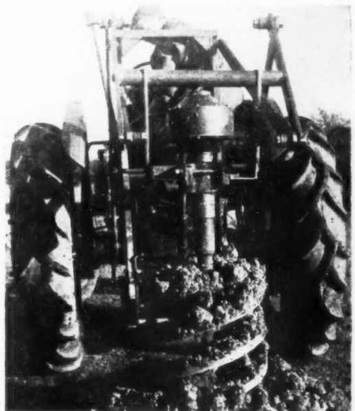
Below, Fig. 1, tractor-operated shovel and back acter.
