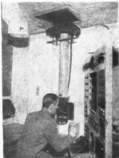
Control panel for heating and ventilation system at the House of Commons; engineer using periscope to see into the new chamber.
