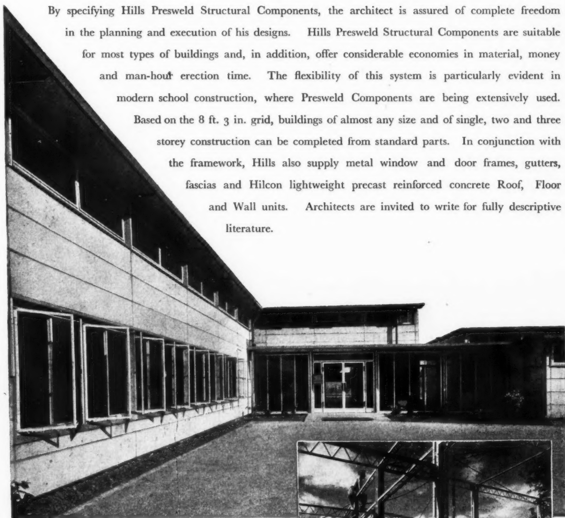
An example of Hills School Construction produced from Hills Presweld Frames, Hills Windows, Window trims and pre-cast reinforced concrete Wall and Roof Units. Junior Mixed and Infants' School, Chessant, Herts. County Architect, C. H. Astin, F.R.I.B.A., M.I.Struct.E.
