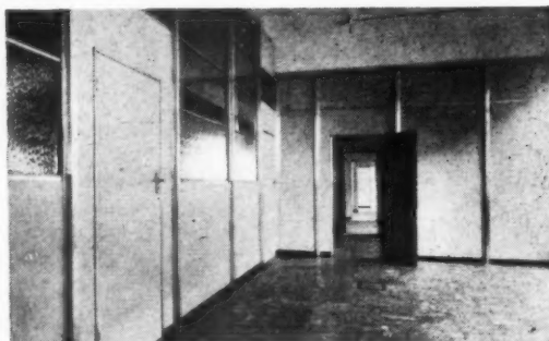
General view of City Offices showing glazed Corridor Partitions 12' high with inter-communicating doors through transverse solid Partitions. Aluminium Junctions and Partitions with 1" cream painted panel..
