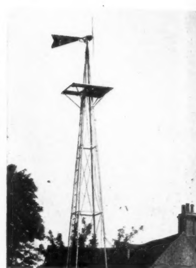
Wind-driven electric generator.
