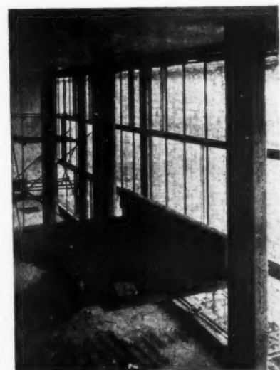
Glazed wall facing Waterloo Bridge. The cantilever staircase is under construction.
