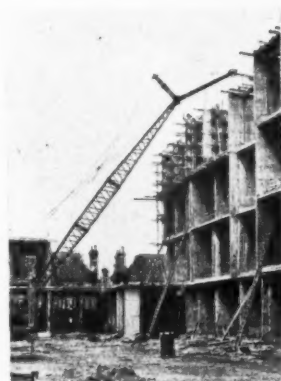
"crane . . . with standard jib of 60 ft. and special swan-neck extension"
