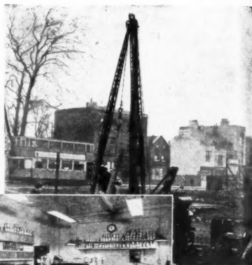
Test boring operations in progress.
