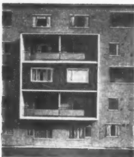
"the protruding elements only extend from the first to the third floors."
