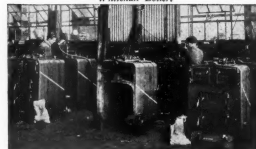
After each unit has passed through the machine shop and been thoroughly inspected, the boiler is assembled section by section for a final test of 100 lbs. hydraulic pressure, and is then dismantled to await despatch.
