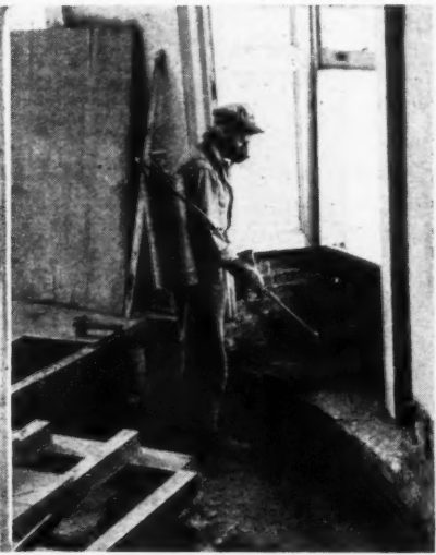
Spraying with Pestcure Dry Rot Solution
