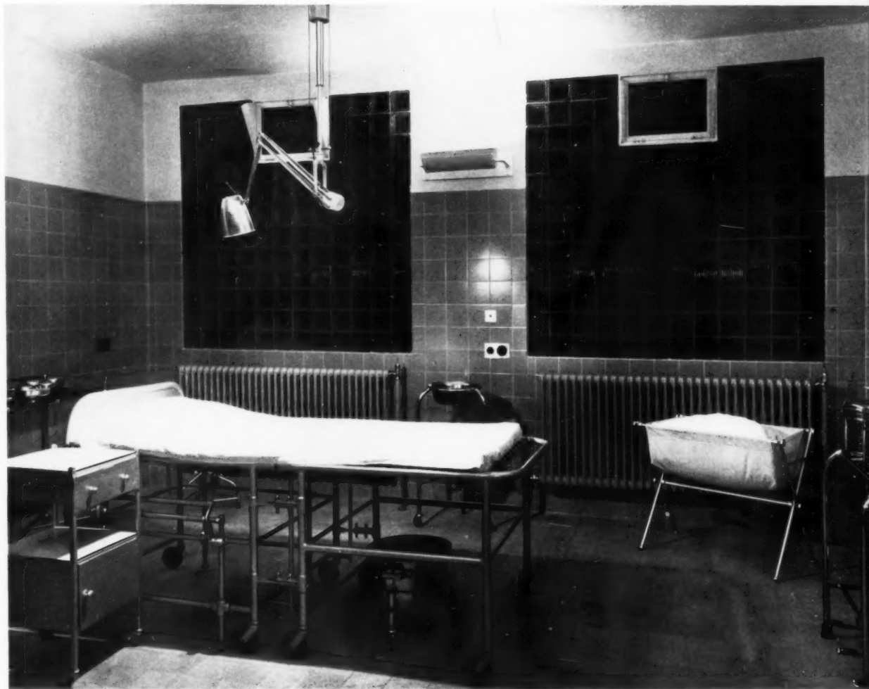
The hopper type opening lights in the glass block panels are in aluminium sub-frames bedded directly on to the glass blocks at sill and jambs.
