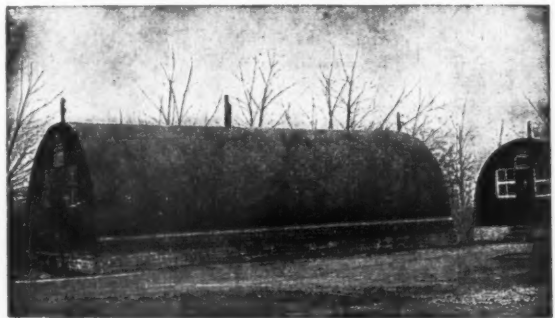
One of the 20 waterproofed Nissen huts at Queen's Park annexe, Chesterfield.
