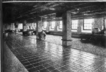
"Consol" steel anchor floor plates in a Dough Room.
