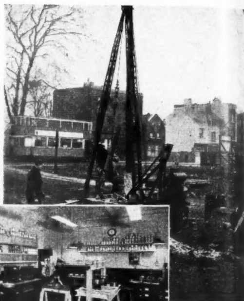
Test boring operations in progress.
