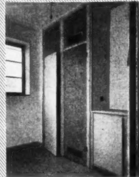
5. 1/2" Pluto Board Panels to cover bathroom water-pipes.
