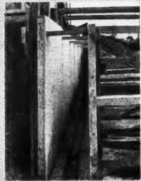
2. 1" Pluto Board bolted to 2 1/2" steel angle frame for concrete shuttering.
