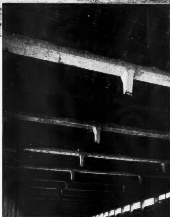
Photograph illustrates the application of 'Fibreglass' quilt under the concrete roof slabs.
