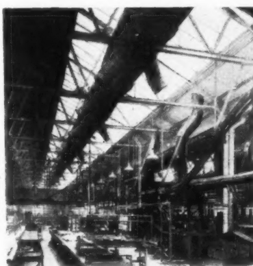
Brightside Plenum Heating in a modern mechanised foundry ; the vitiated air is extracted and replaced by warm clean air. The smaller illustration shows a plenum installation in a machine shop.
