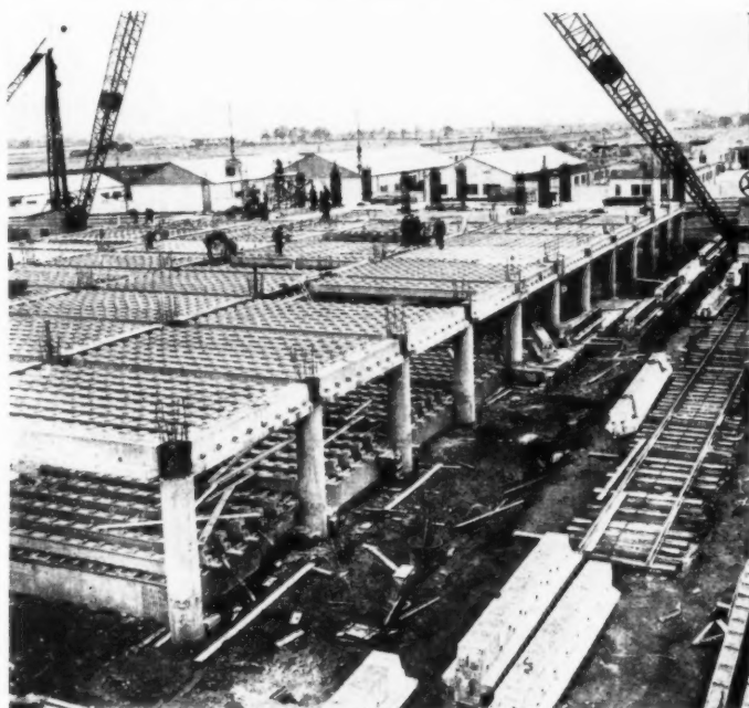
Top, left, warehouse for HMSO, Sighthill, Edinburgh. Above, the first floor with prestressed concrete beams on cylindrical columns of normal R.C. and columns to second floor commenced. Below, typical details of floor beams. (See 19.118). Illustrations—Crown Copyright Reserved.
