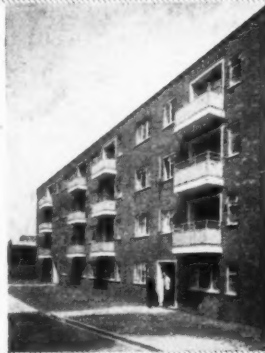
1. 1" Pluto Board Balcony panels screwed to mild steel frame.
