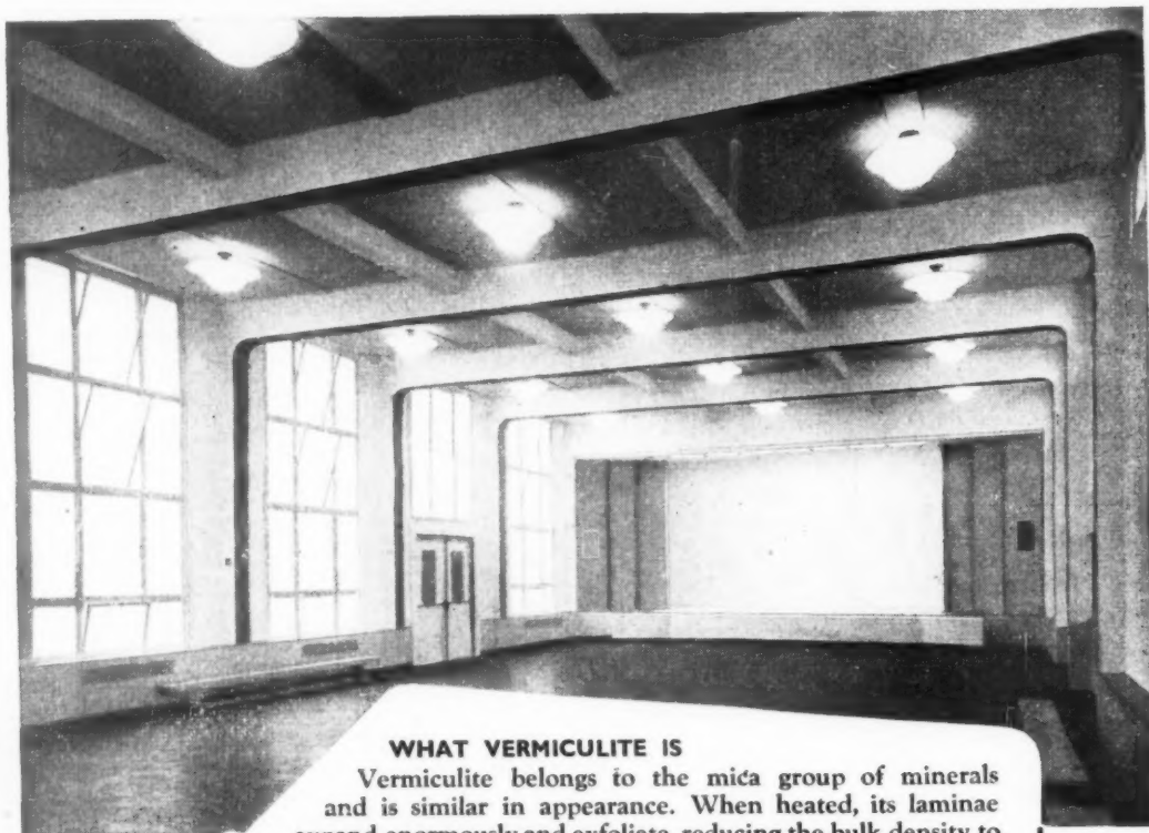
"Kisol" Vermiculite Plaster for inside wall and roof treatment for London County Council School.
