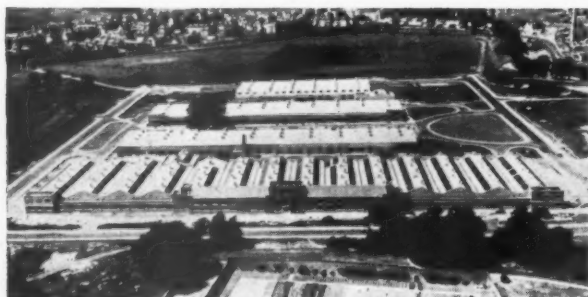
VALE OF LEVEN ESTATES. Base concrete floors waterproofed with EVODE MELLITOL incorporated in the mix and granolithic finish hardened and dustproofed with EVODE PROVER II Surface Treatment. Consulting Architects: Messrs. Wylie, Shanks & Wylie, Glasgow. Co-ordinating Surveyors: Messrs. W. & J. R. Watson, Ltd., Edinburgh. Published by courtesy of Scottish Industrial Estates Ltd.
