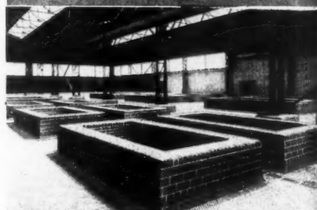
Acid Resisting floor in a Galvanising shop.
