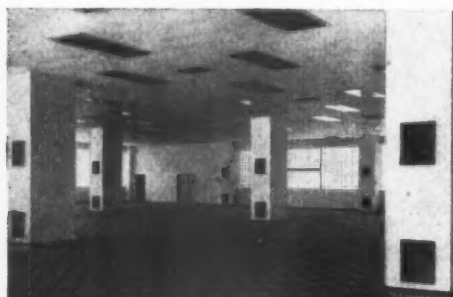
Red "Ferrogan" flags on concrete base in Printing Works.
