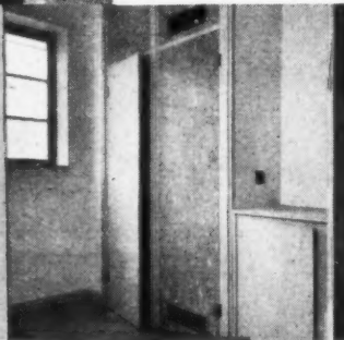
2. Balcony Panels made from \frac{1}{2} " Pluto Board and screwed to mild steel frame.
