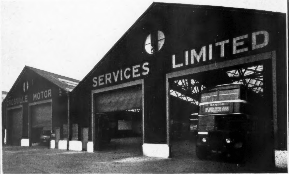
Messrs. Crosville Motor Services, Ltd., Bangor, North Wales Garage, fitted with 4 Kinnear Shutters, each 15' 7" high x 16' 2" wide.
