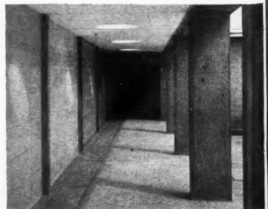
Below, under the covered way, looking east; note the tooled finish to the columns.
