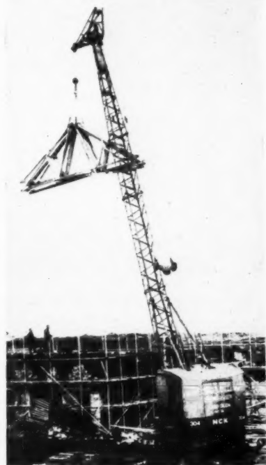
Fig. 8. Crane carrying roof trusses.
