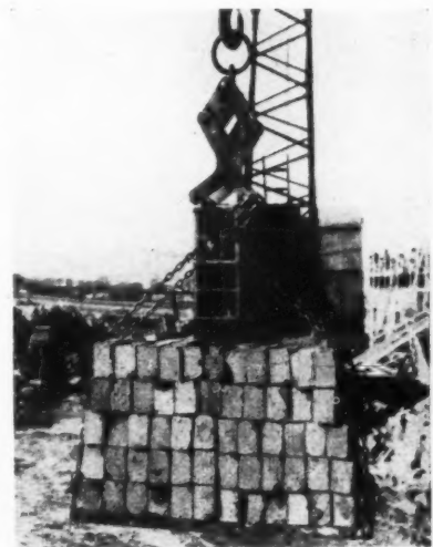
Fig. 3. Brick sling being handled by crane.
