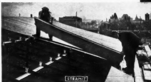
(Below) Precut STRAMIT 2in. roofing slabs approximately 9ft. 6in. by 2ft. are laid in STRAMIT 18G Steel Tees and are held down by standard STRAMIT clips. The slabs' ends are supported on the purlins. This portion of roof will be copper covered—other parts will be felted.
