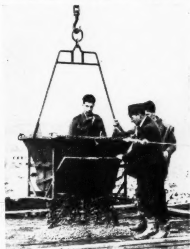
Fig. 7. Hopper discharging concrete.
