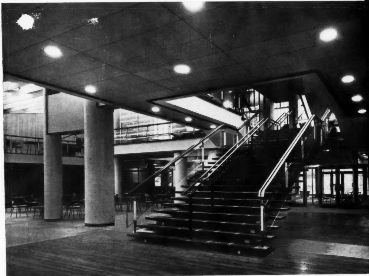
Panels of toughened glass are held by bronze brackets between the anodised aluminium - and plastic - covered tubular metal balusters: the handrail is in mahogany.
