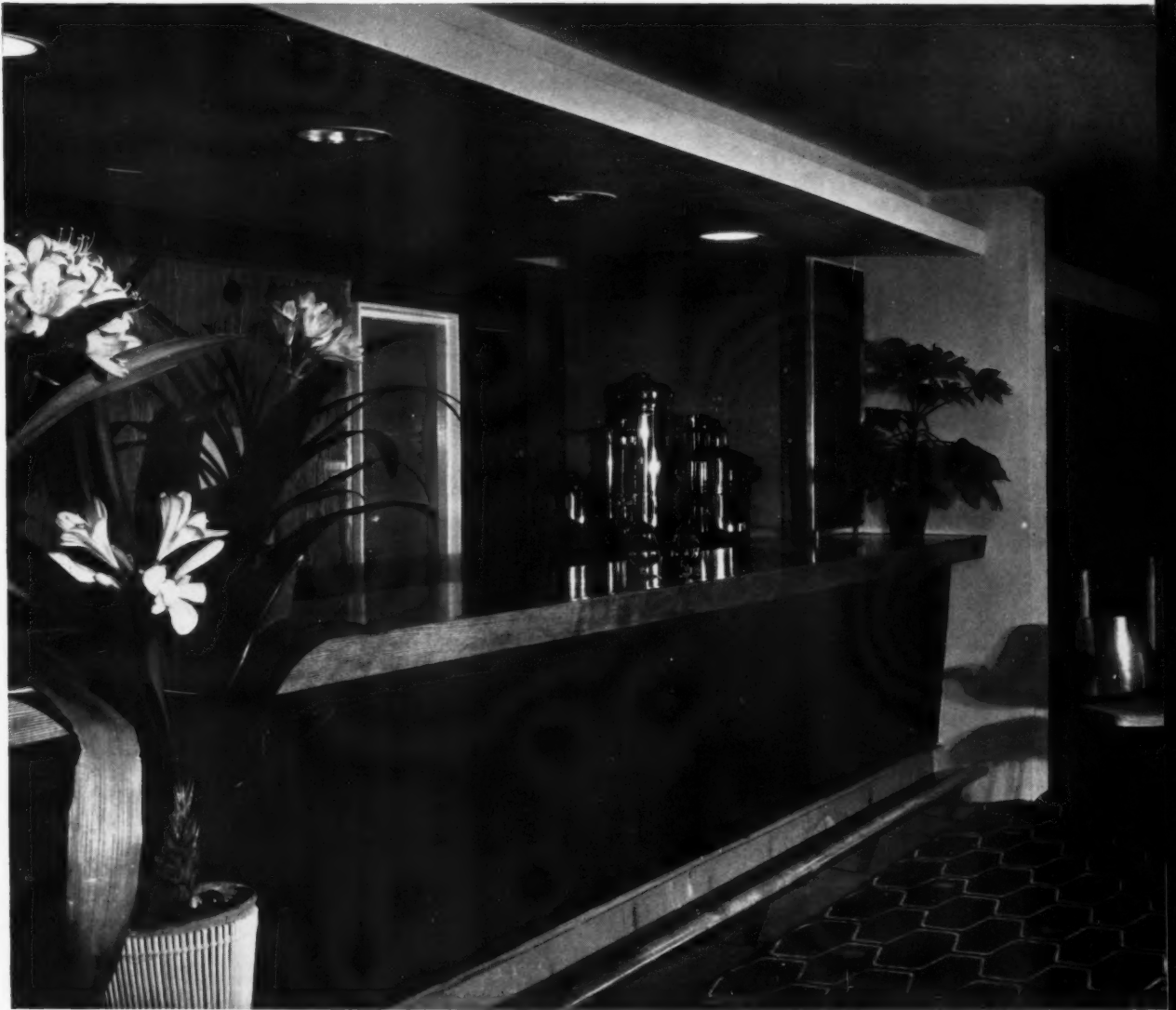
The counter front is of finely corrugated enamelled aluminium : the fitting behind is veneered in ash.
