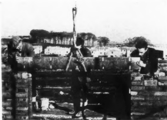
Left, Fig. 5, crane lowering lintol.
