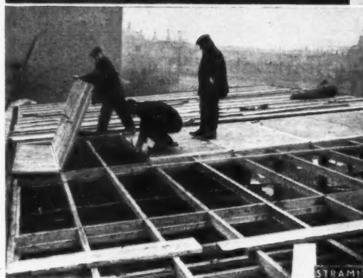
(Top left) Illustration showing A TYPICAL EXAMPLE OF STRAMIT PARTITIONING erected for the British Electricity Authority in London.
