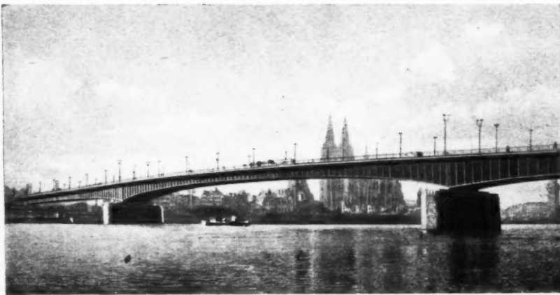
The new Rhine bridge at Cologne-Deutz. Riveted plate girders, continuous over the river piers, with a centre span of 605 ft. See 20.196.
