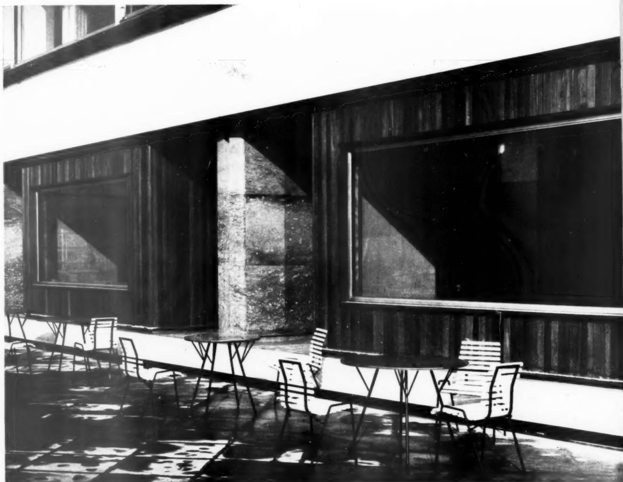
The outside walls of the bay are faced with vertical teak strips and the window, which is a single sheet of polished plate glass in a teak frame, has flower boxes on the restaurant side.
