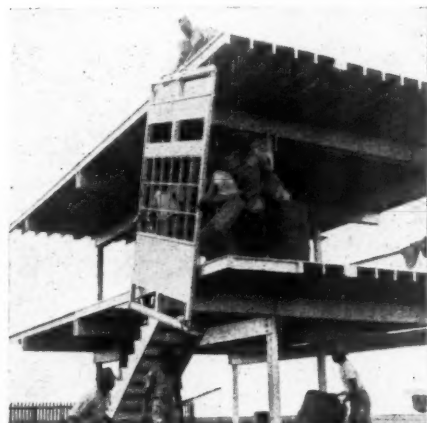
First wall panel being raised.
