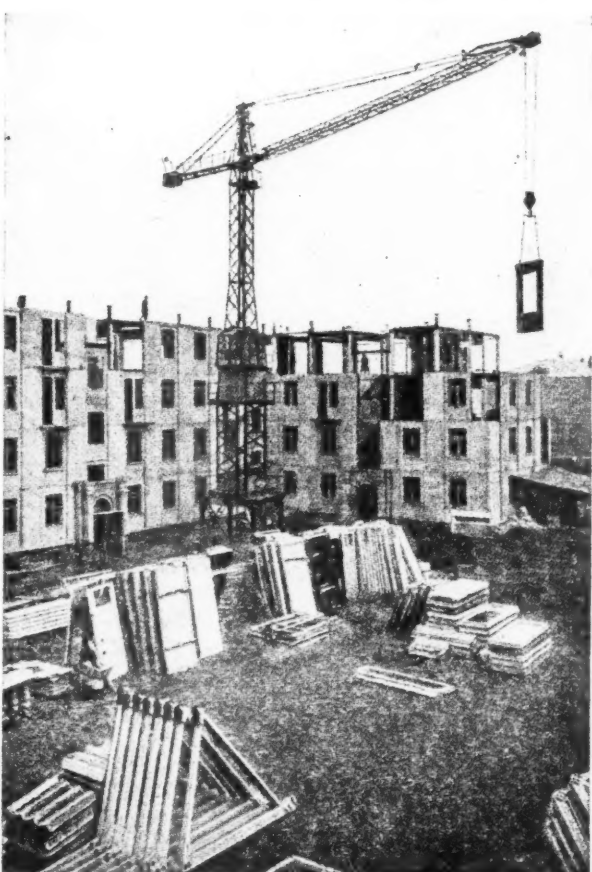
Fig. 2. Tower crane lifting pre-fabricated window unit into position on multi-storey block of flats. Note tidy stacks of other prefabricated units in foreground.
