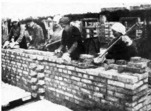
Fig. 1. Team of five bricklayers at work. The woman on the right is using a long-handled trowel.
