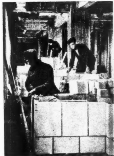
Above, Fig. 4, a covered gantry in use on the block of flats being erected on the Kotelnicheskaya Embankment in Moscow. The gantry has reached the top of the main, 17-storey section of the building, which contains, on the ground floor, a departmental store and on the upper floors, 700 one-, two-, three-, and four-room flats. Below right, Fig. 5, men working inside the gantry.
