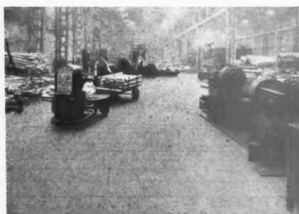
"Ferrogran" Flag flooring in heavy Extrusion Mill.
