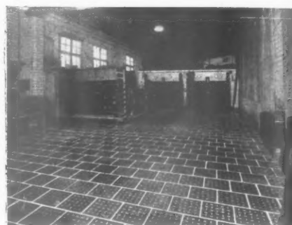
"Consol" plate flooring in a Bakery.
