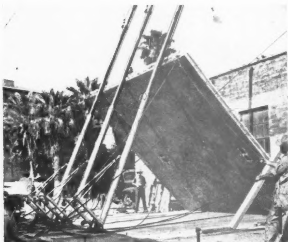
Raising a 22-ft. concrete wall slab.
