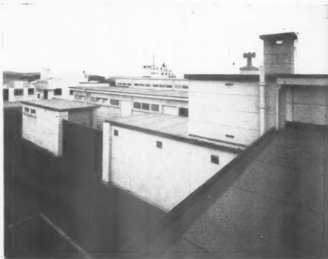
Roof of Ronaldsway Airport, I.O.M. screeded with "KISOL" Vermiculite.
