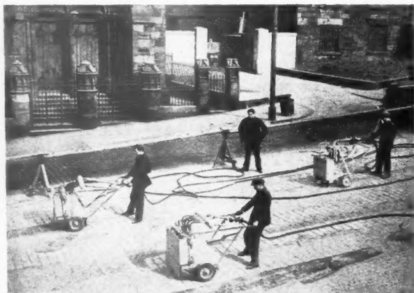
The use of pneumatic machines for roughening the surface of a road which has worn smooth.
