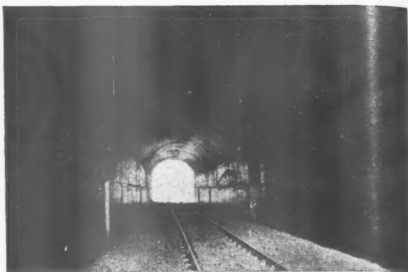
By Permission of British Railways. Railway Tunnel at the Consett Iron Co., Ltd., Durham. Internal concrete surface painted with EVODE PROTECTIVE (Chlorinated Rubber) PAINT. Consultants: Messrs. International Construction Co., Ltd., 56 Kingsway, London, W.C.2. Contractors: Messrs. F. C. Construction Co., Ltd., City Road, Derby.
