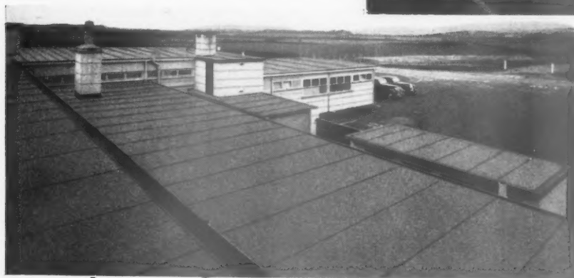
Roof of Ronaldsway Airport, I.O.M. screeded with "KISOL" Vermiculite.
