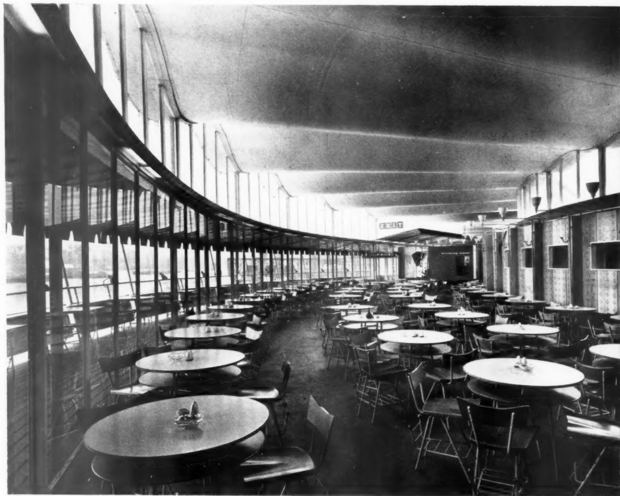
The undulating roof is composed of two skins of sheet aluminium with a filling of cork.
