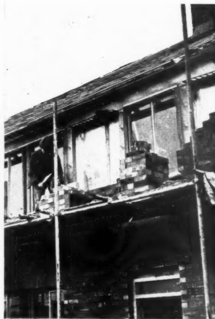
Above, Fig. 11, the prefabricated shell complete and weatherproof.
