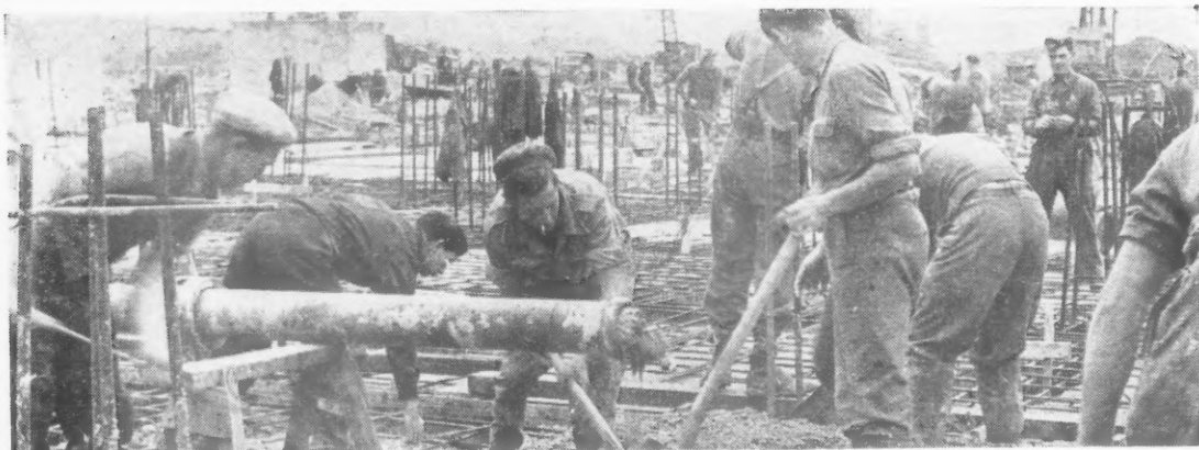
Concrete pumped by pipeline
