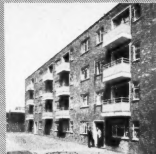
5. \frac{1}{2} in. "Pluto" Board Balcony Panels screwed to mild steel frame.
