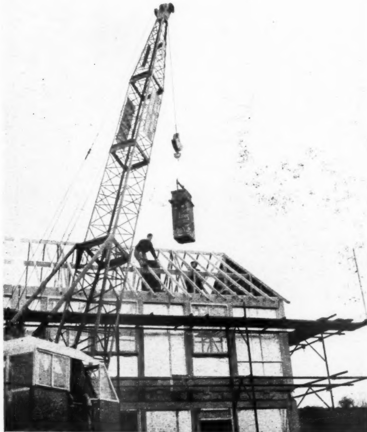
Fig. 16. Top section of chimney, built at ground level, being hoisted into position by mobile crane.
