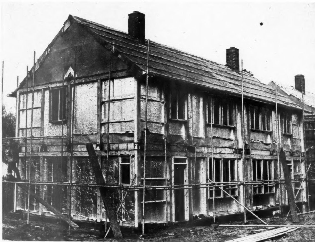
Above, Fig. 11, the prefabricated shell complete and weatherproof.
