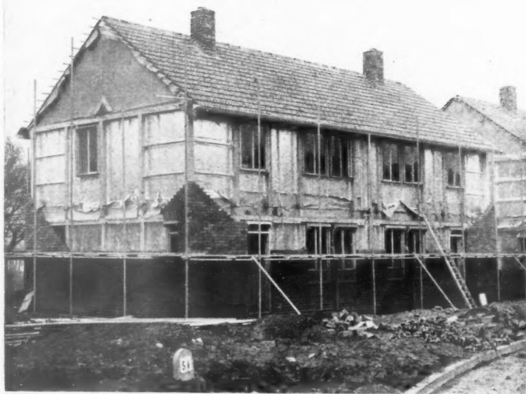
Above, Fig. 12, tiling completed (except end courses) before brickwork commenced. Right, Fig. 13, brickwork nearly completed. (N.B. No further scaffolding required; chimney has already been placed in position by crane.)
