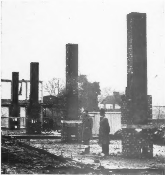
Three stages in the erection of the prefabricated shell. Left, (Fig. 2), the foundation slab and the free-standing chimneys. Below left (Fig. 3), the ground floor wall units and the floor panels. Below right (Fig. 4), the first floor wall and partition units.
