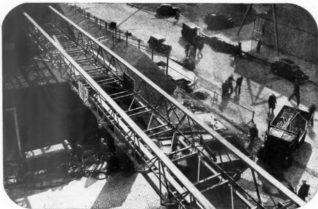
WELDED TUBULAR BRIDGE BETWEEN "MINERALS OF THE ISLAND" AND "POWER AND PRODUCTION" BUILDINGS.
