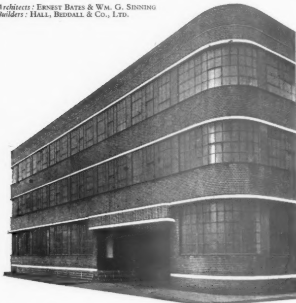
By courtesy of BRITISH TROLLEY TRACK CO., LTD. Factory at Copperfield Street, London, S.E.1, showing excellent example of slate cill and window board with slate facings between windows.
