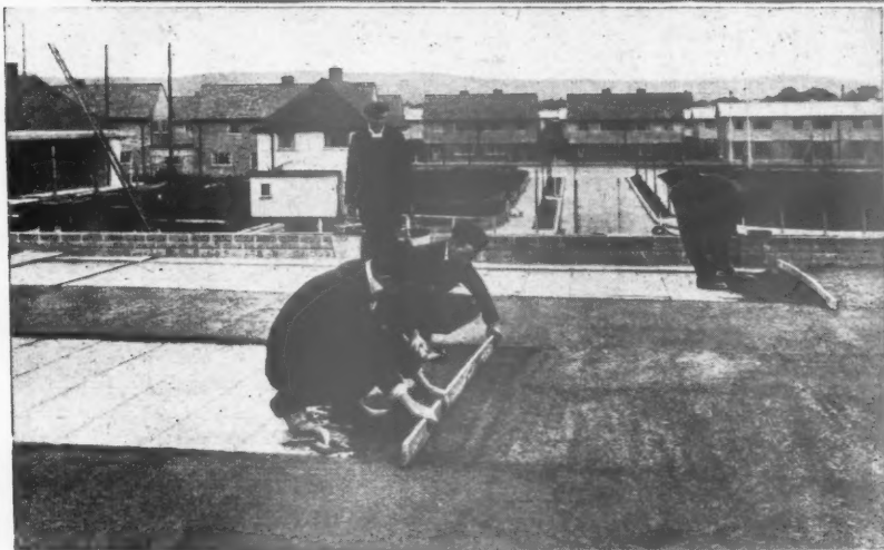
KISOL Vermiculite ready mixed screed being applied to the roof of Gabalfa School, Cardiff.
