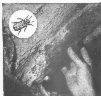
A rosette in the roof of Chichester Cathedral showing damage by the Death Watch Beetle.
