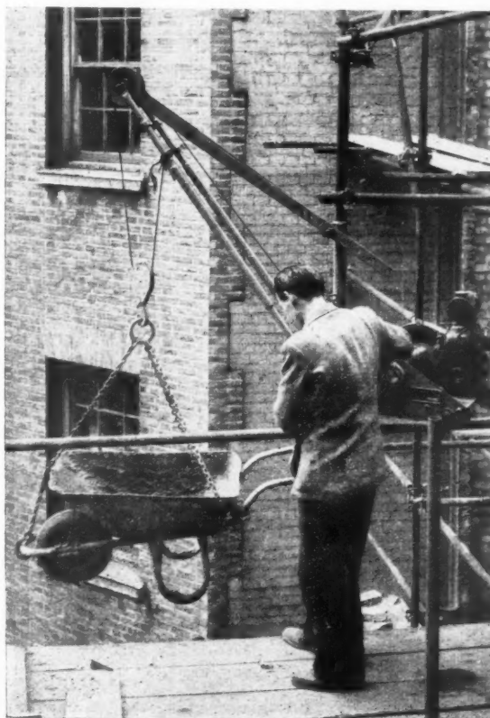
Fig. 7. Power-operated gin-hoist mounted on swivelling bracket fixed to the scaffold, so that the load can be swung in and placed on the scaffold.
