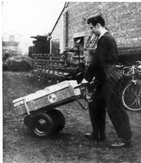
Fig. 6. Special brick barrow for use with hoist shown in Fig. 5. This will pick up, wheel and deposit in a neat stack, 40-50 bricks at a time.
