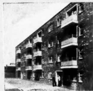
5. 1/2" 'Pluto' Board Balcony Panels screwed to mild steel frame.
