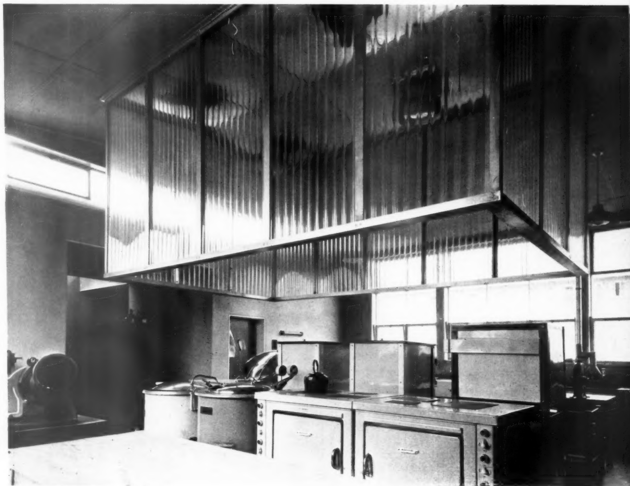
The sides of the hood are panels of corrugated transparent plastic sheeting held in metal sections and the top is lined with aluminium sheeting on fibreboard.
