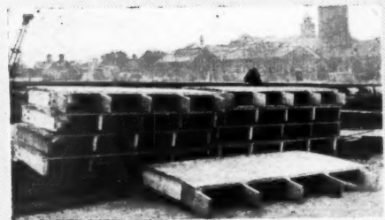
2. 'Pluto' Board used for circular shutters, oiled and ready for erection.
