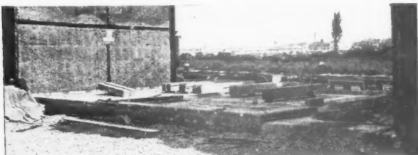
The brick base before shuttering is erected.
