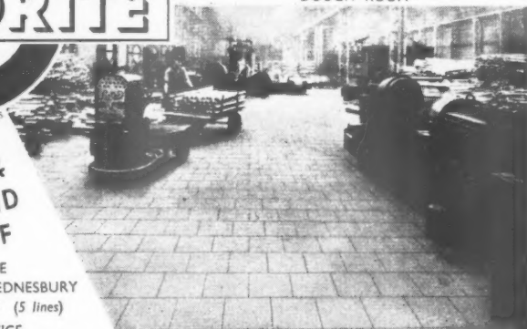
FERROGRAN FLAG FLOOR IN HEAVY EXTRUSION MILL
