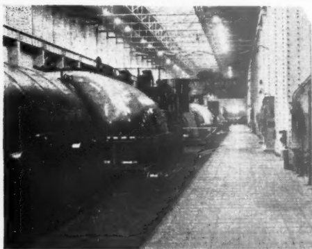
RED PRODORDUR TILE FLOORING IN TURBINE HOUSE OF NORTHERN POWER STATION
