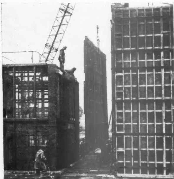
Shuttering being placed in position.
