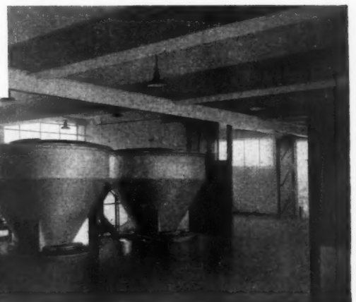
ACID RESISTING POLISHED ASPHALT FLOOR IN FRUIT ESSENCE FACTORY
