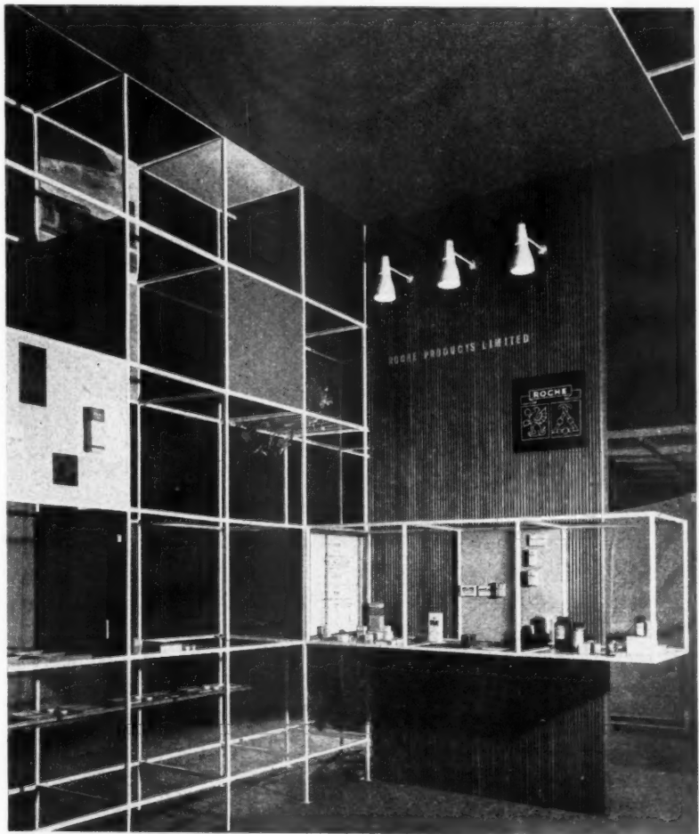
The stand for Roche Products, Ltd., at the recent London Medical Exhibition was designed by Ian Bradbery. The site was 16 ft. by 12 ft., open on three sides, and consisted of a space frame, seen in the photographs above and below, five display
