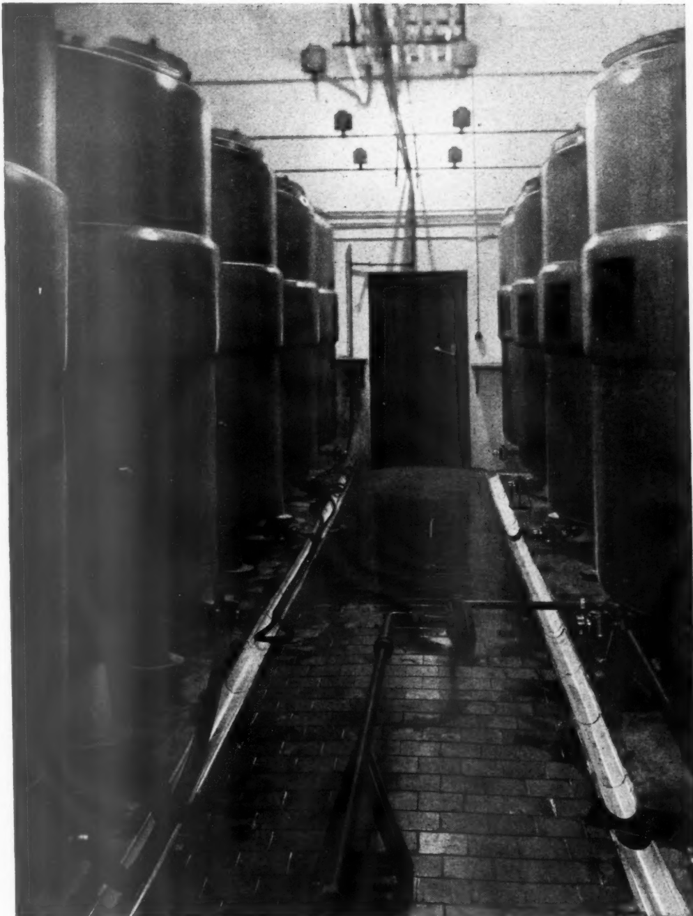
Wheatly Quarry Tile Floor in the Cooling Room of the Uganda Breweries Ltd. at Port Bell
