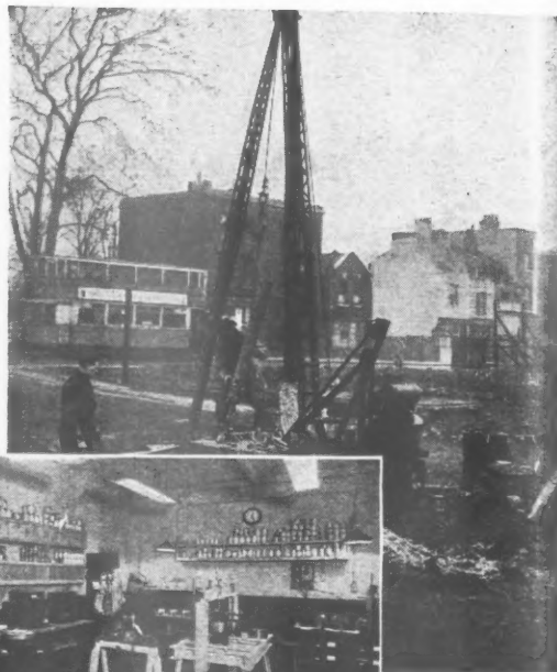
Test boring operations in progress.
