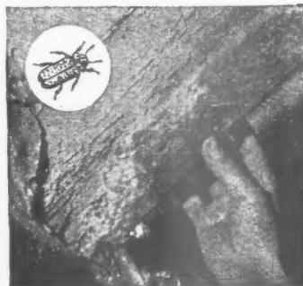
A rotter in the roof of Chichester Cathedral showing damage by the Death Watch Beetle.
