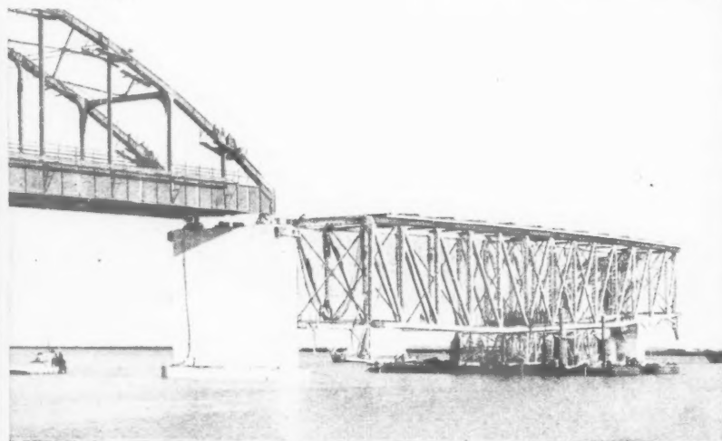
Vila Franca bridge under construction, showing (on right) the service span used as a temporary support when erecting the permanent steelwork.
