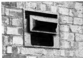
The terminal can be fitted even in proximity to overhanging, or other projections. There is no flue pipe or cowl.
